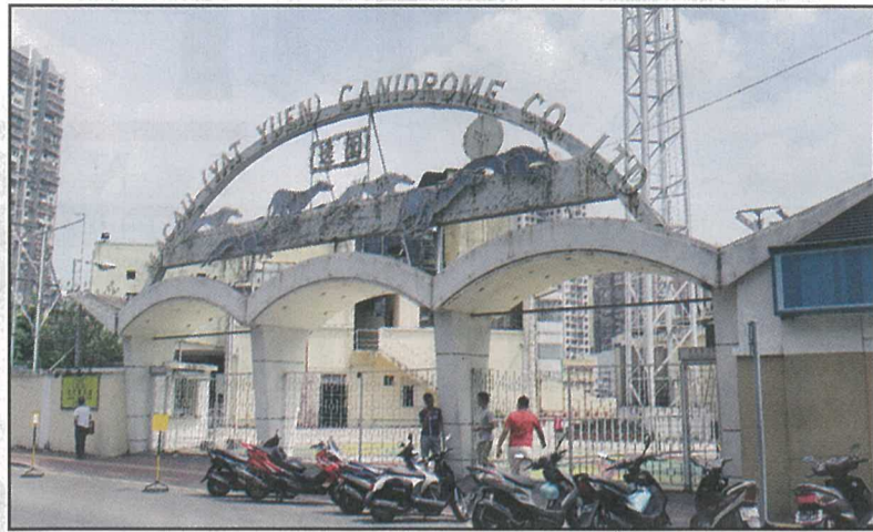
Pedestrians walk past Yat Yuen Canidrome in Fai Chi Kei yesterday.
