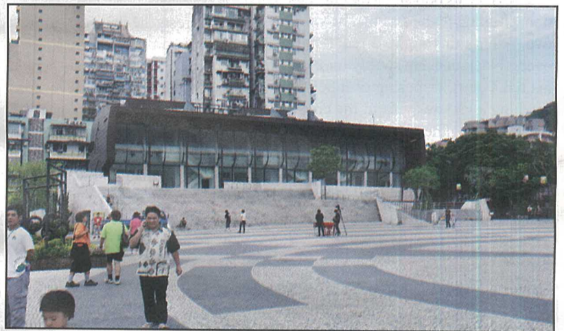
Pedestrians walk past the leakage-hit Tap Seac Commercial Centre (commonly known as "Tap Seac Glass House") in Praça do Tap Seac yesterday.
