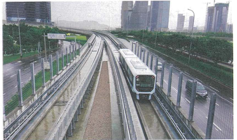
This undated photo taken from the website of the Transport Infrastructure Office (GIT) shows a Light Rail Transit (LRT) train during tests near Ocean Gardens in Taipa in June.
